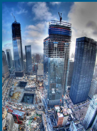
WTC In Progress March 2012
