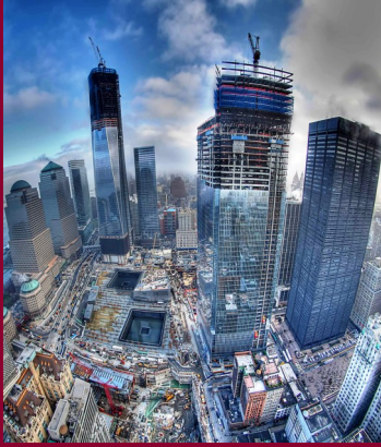
WTC In Progress March 2012
